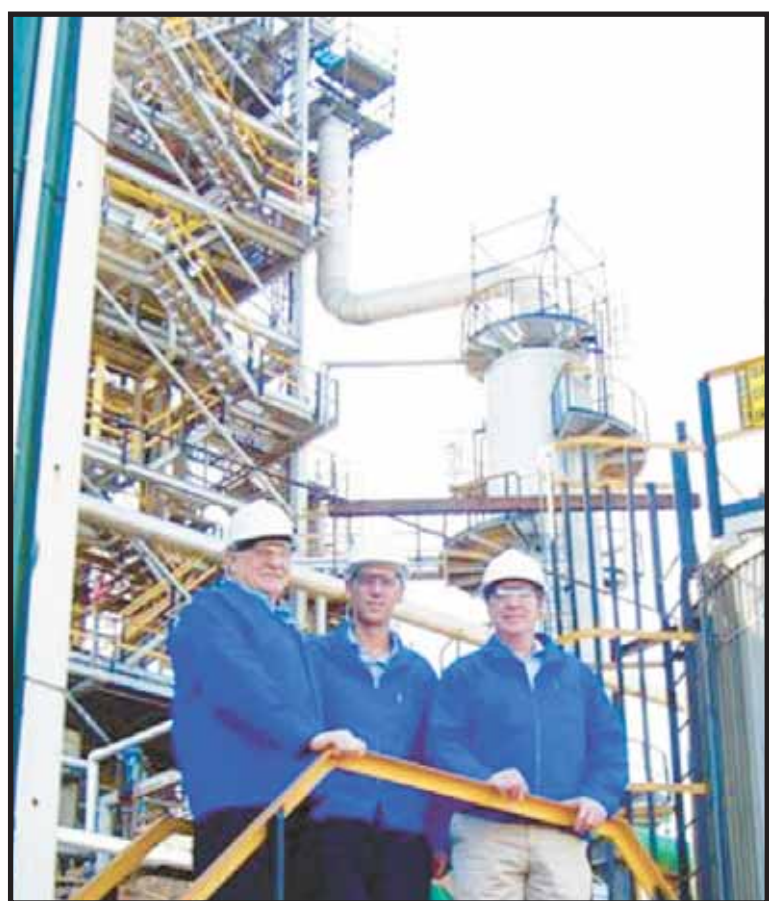
Pictured in front of the new imported reactor at Isegen are, from left, the company's three shareholders: Robert Fowlds, managing director; Mark Holtes, marketing director; and Paul Tack, operations director.
